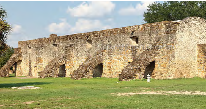
MISSION SAN JOSE BUTTRESSES AND MASONRY
