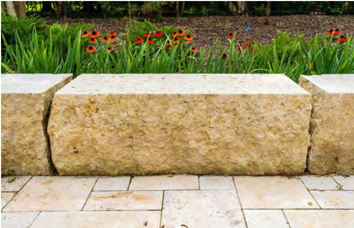
LIMESTONE BLOCK SEAT WALLS
